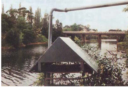
The Nepean River, as seen from the pump house on the eastern bank servicing Kirkham Estate.
